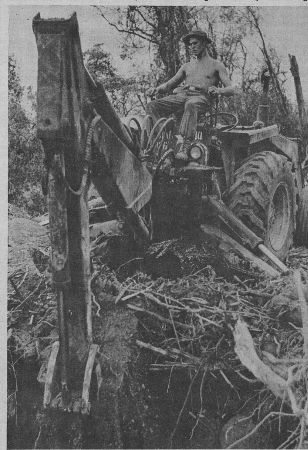
The backhoe, brought in by air, is put to work gouging out a command bunker.
