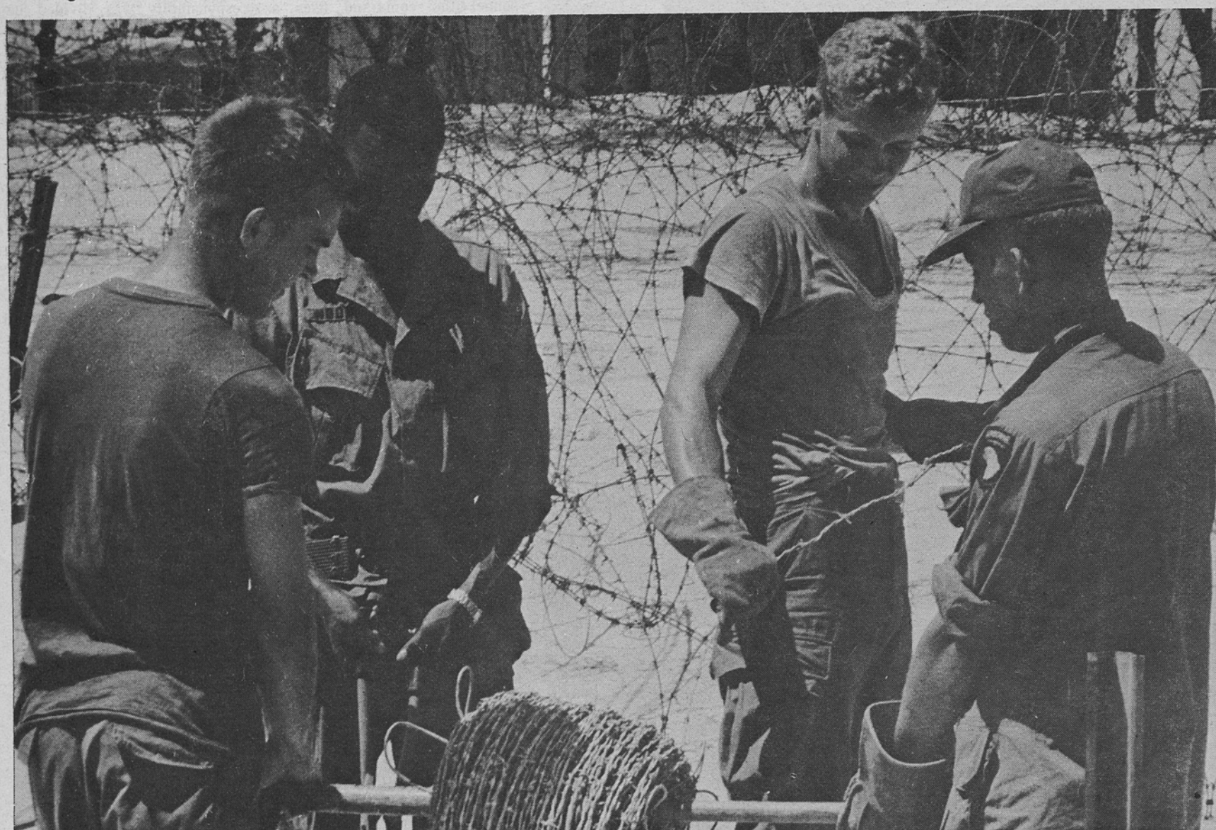
"Screaming Eagles" from the 326th Engineer Battalion string barbed wire around the perimeter of a recently built fire support base east of Hue.
