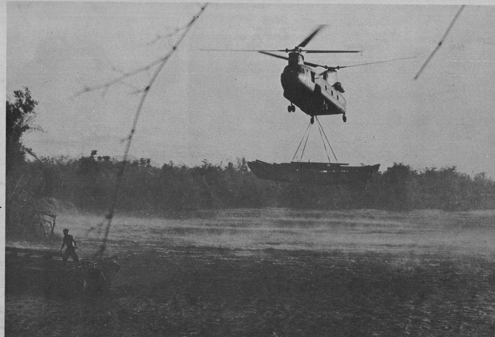
When speed and power are of the essence, the engineers must call on the versatile Chinook as they do here in floating a section of pontoon bridge.
