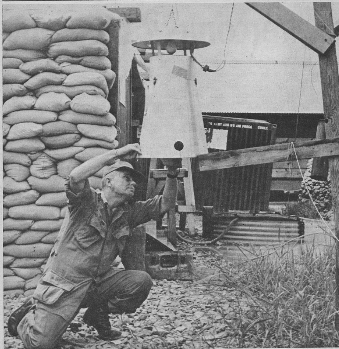
Mosquitos are trapped in this "New Jersey Light Trap" and then removed for inspection.
