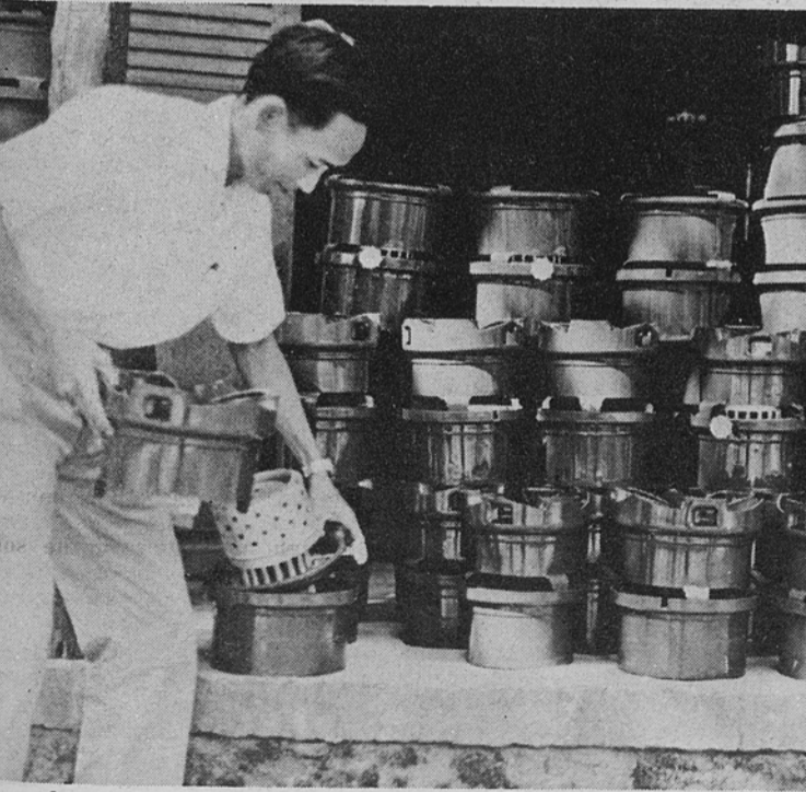
A member of the Labor Office installs the wick mechanism into the base of a stove.
