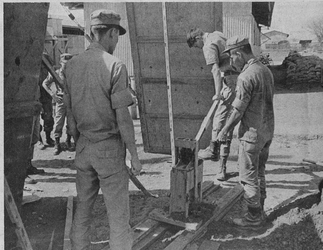
Medical battalion soldiers make bricks from sand and cement for new medical building.
