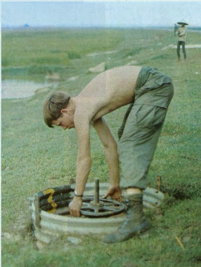
Opening the valve starts the fuel pumping.
