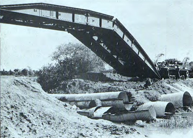
Sometimes, the divisional engineers are called upon to bridge a river immediately. They usually solve the problem with Armored Vehicle Launched Bridge (AVLB).
