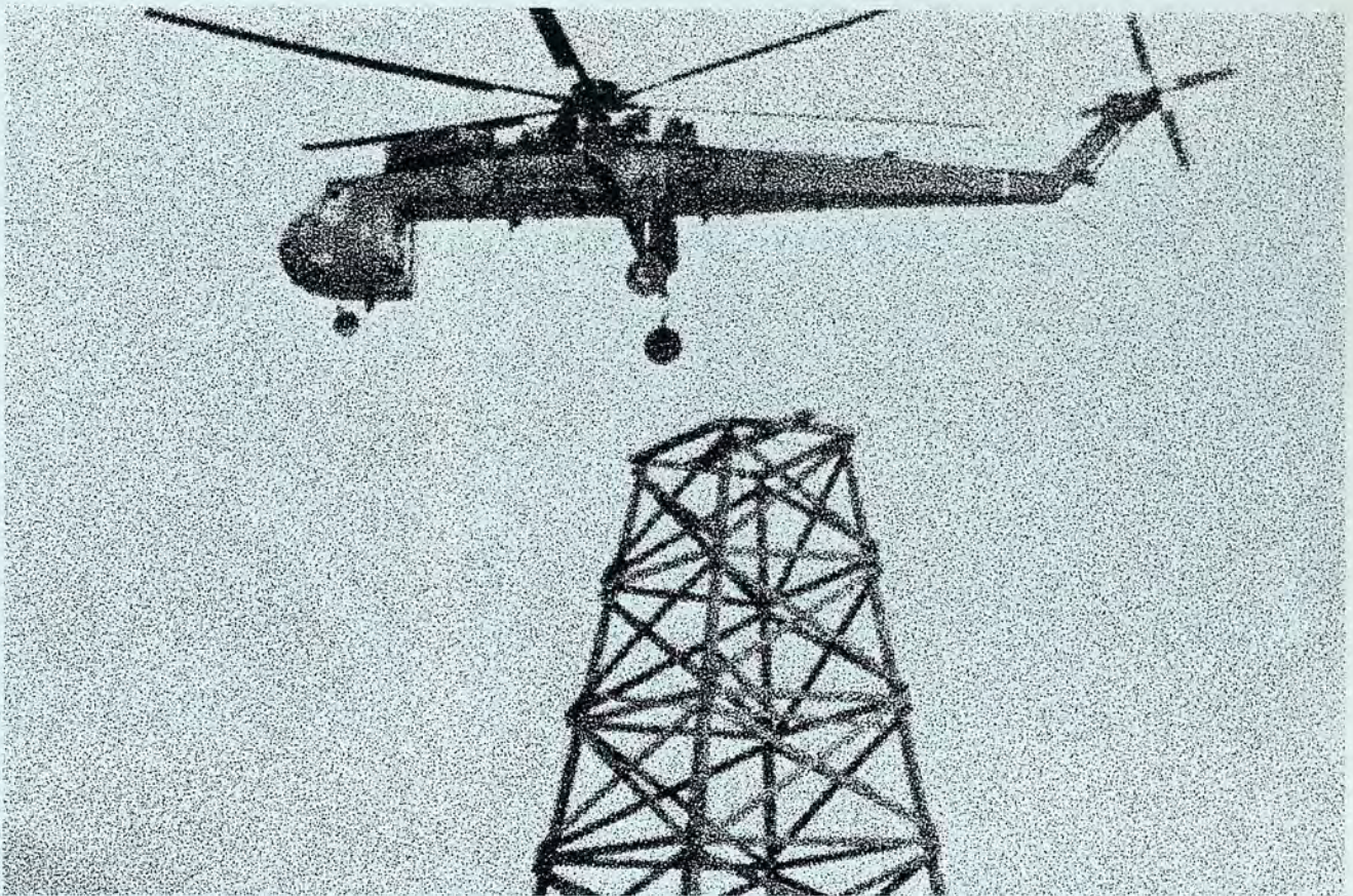
Once the observation tower was completed, an Army CH-54 Sky Crane was called in to lift it into place.
