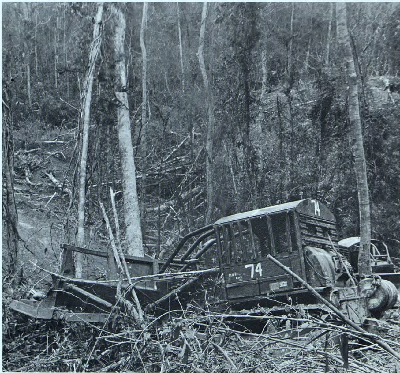
The ARVN engineers worked along with their American counterparts in operating the Rome plows.
