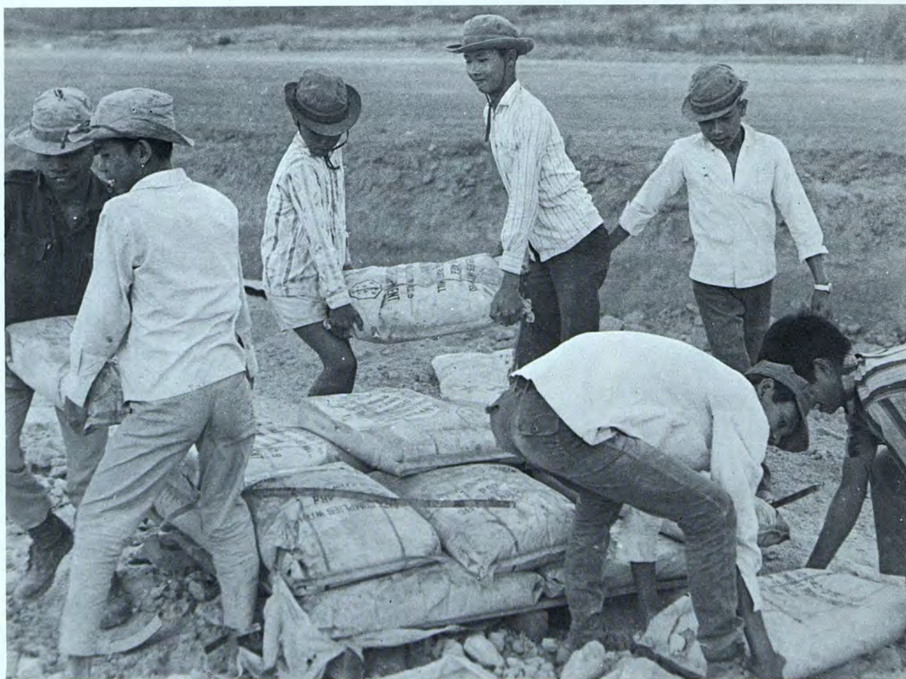
The work continued on QL-13 as the cement bags were distributed over the roadbed.
