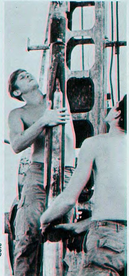
The drill tool extension is lowered through the casing (below) and is then attached to the drill stem (left).
