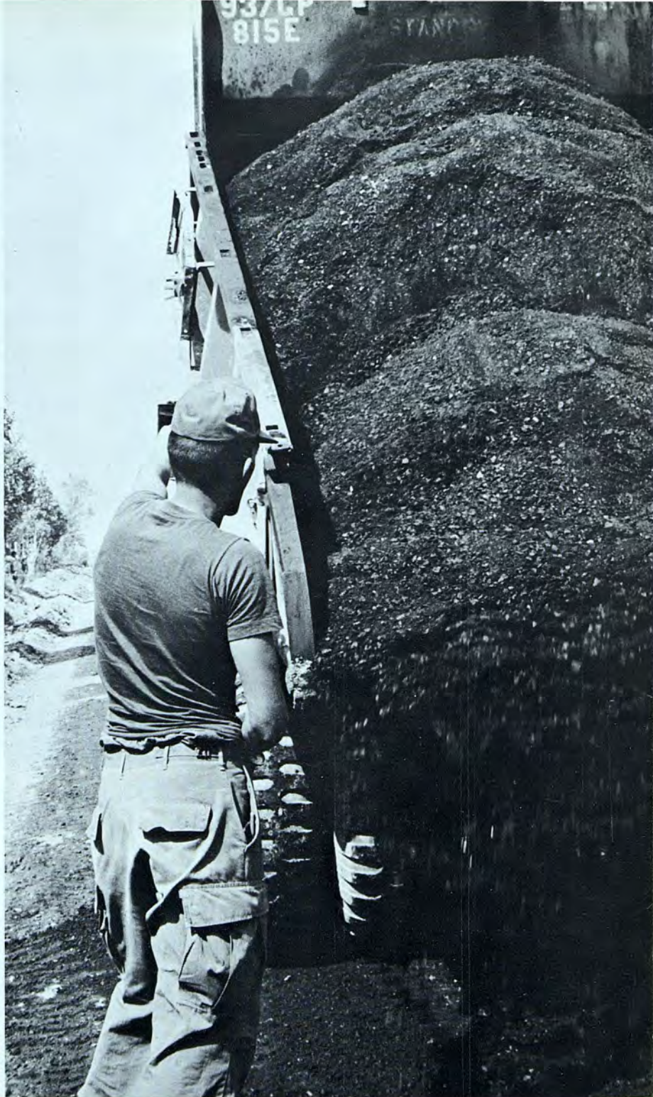
After the cold mix asphalt is dumped, spreading and compacting are the two remaining steps.
