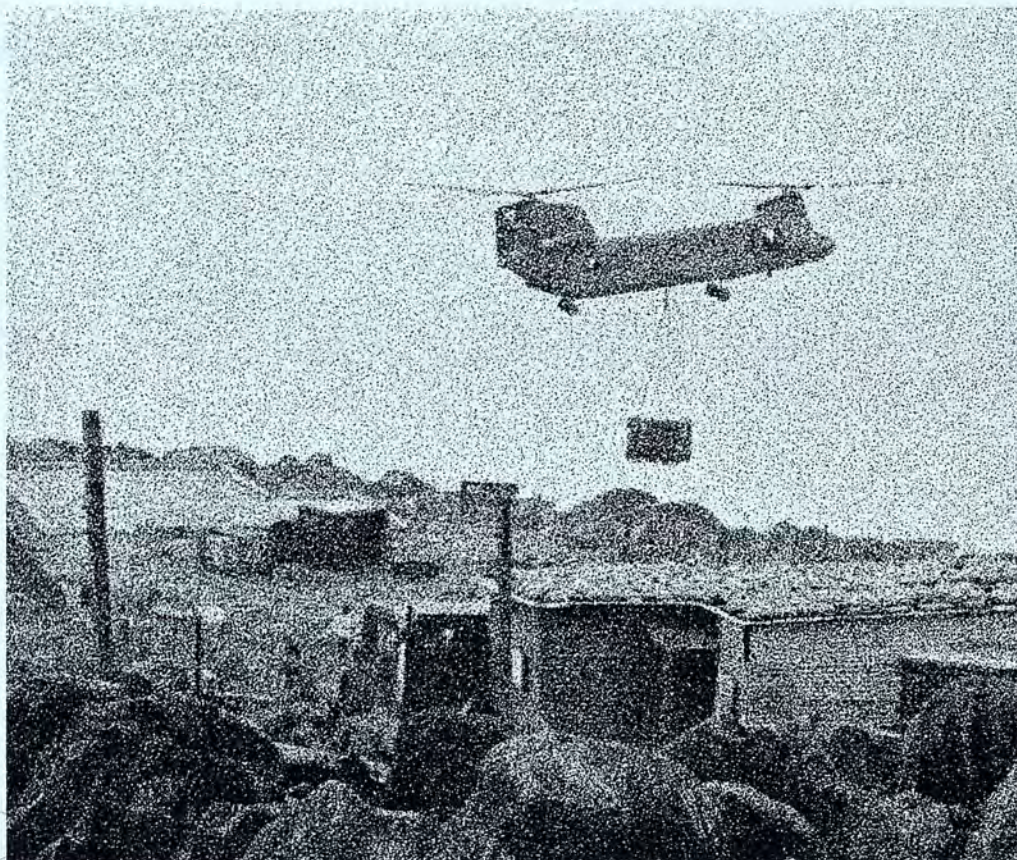
A Chinook helicopter airlifts ready-mix concrete to the summit of Nui Ba Den.
