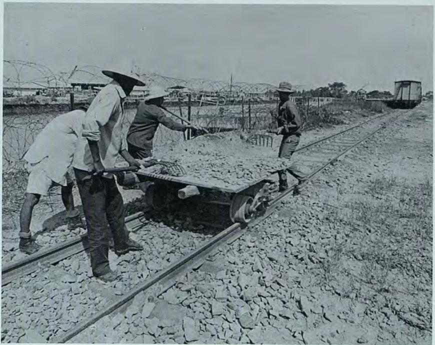
*National Vietnamese Railway workers patch the roadbed on a rail that once ran uninterrupted from Saigon northward to Hanoi and China (above). Twenty-five tons of gravel pour out of a hopper car at the end of the line—Xuan Loc (below)*
