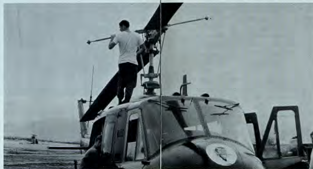
A Devil ship has its hydraulic dampers checked.
