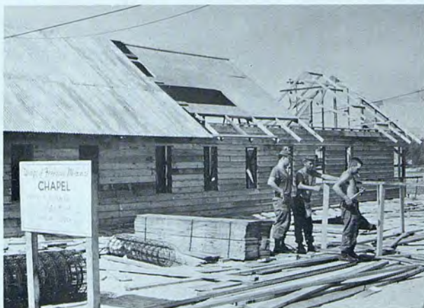
Three volunteers work on forms for the roof of the chapel.
