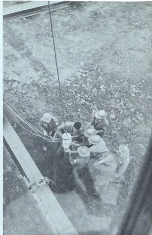
ARVN engineers attach the big hook to a 9,000 pound beam.
