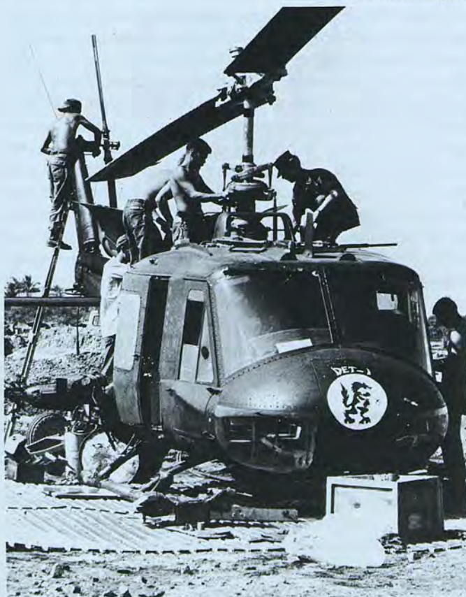
Maintenance crew pours over a Det 1 UH-1B in early 1968. These war-weary helicopters took a lot of TLC and Navy ingenuity to keep operational. (Via Bell Helicopter)
