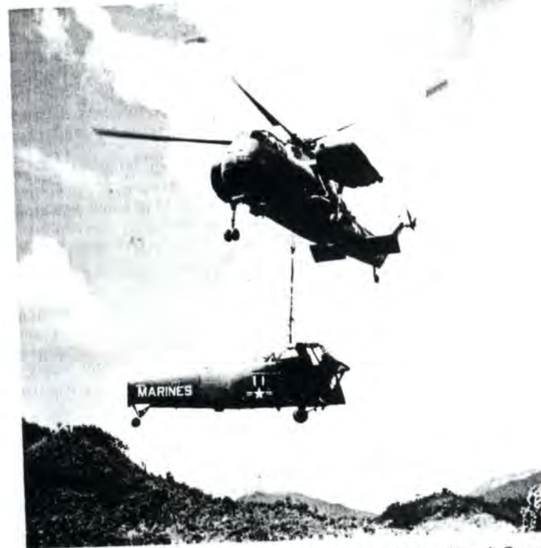
It took two days, with a battle raging nearby, for a Marine Aircraft Group (MAG)-16 maintenance crew to dismantle a troop-carrying UH-34D helicopter so that a larger CH-37 could carry it home. This action took place within ten miles of Danang in October 1965.
