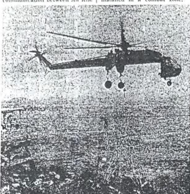
**EASY DOES IT**—A Flying Crane from the 458th Aviation Company gently lowers an antenna tower to its cement pad atop Hon Cong mountain overlooking Camp Radcliff at An Khe. The tower is part of a communications system linking An Khe to the Qui Nhon area.
