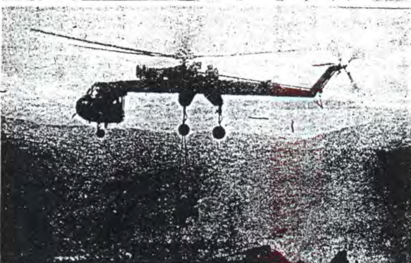
BIG LIFT —A giant Skycrane moves away with a bulldozer in tow after the 4th Engineers had cleared another 1st Brigade firebase in the dense jungle near Dak To.
