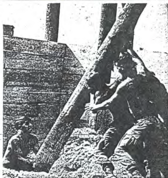
173rd Abn Photo MEMBERS OF THE 173rd Engineers, 173rd Airborne Brigade use brute strength to seat a pole for the foundation of a new operations building near Bong Son.
