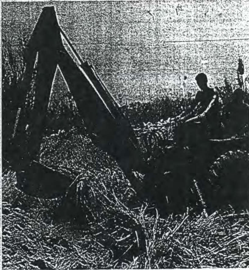
TWO SOLDIERS from the 8th Eng. Bn., 1st Air Cav guide the crooked arm of a backhoe digger scooping out new bunkers at Landing Zone Carolyn. The soldiers completed two landing zones in a two-week period.
