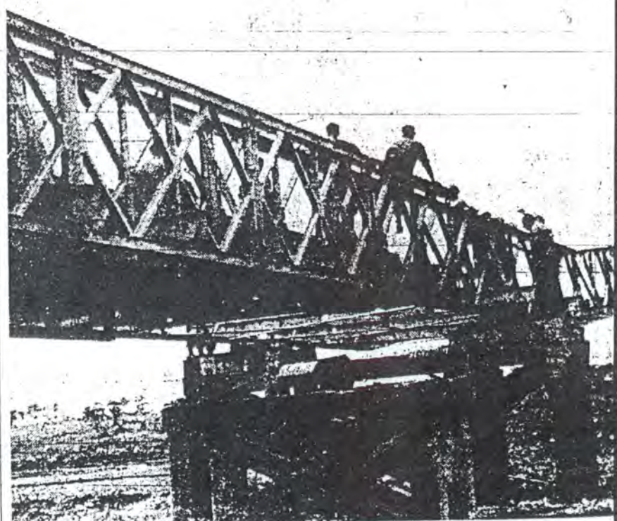
TIME OUT —Reaching the mid-way point of its cautious yet steady journey Suoi Cai River, this bridge structure is temporarily halted to allow adjusting the center pier. The bridge is being built by Company B, 1st Engineer Battalion (Photo by PFC Robert J. Stevens, 1st Infantry Division).
