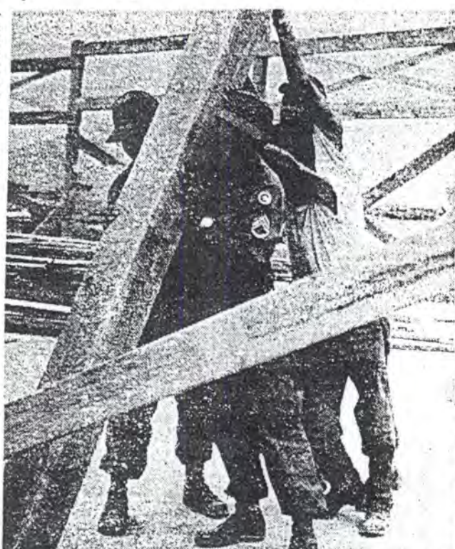
HEAVE HO!—Four men from the 553rd Engineer Detachment raise a section of a prefabricated building being constructed to serve as a ration breakdown center for the 196th Infantry Brigade. (Photo by 1st LOG-10)
