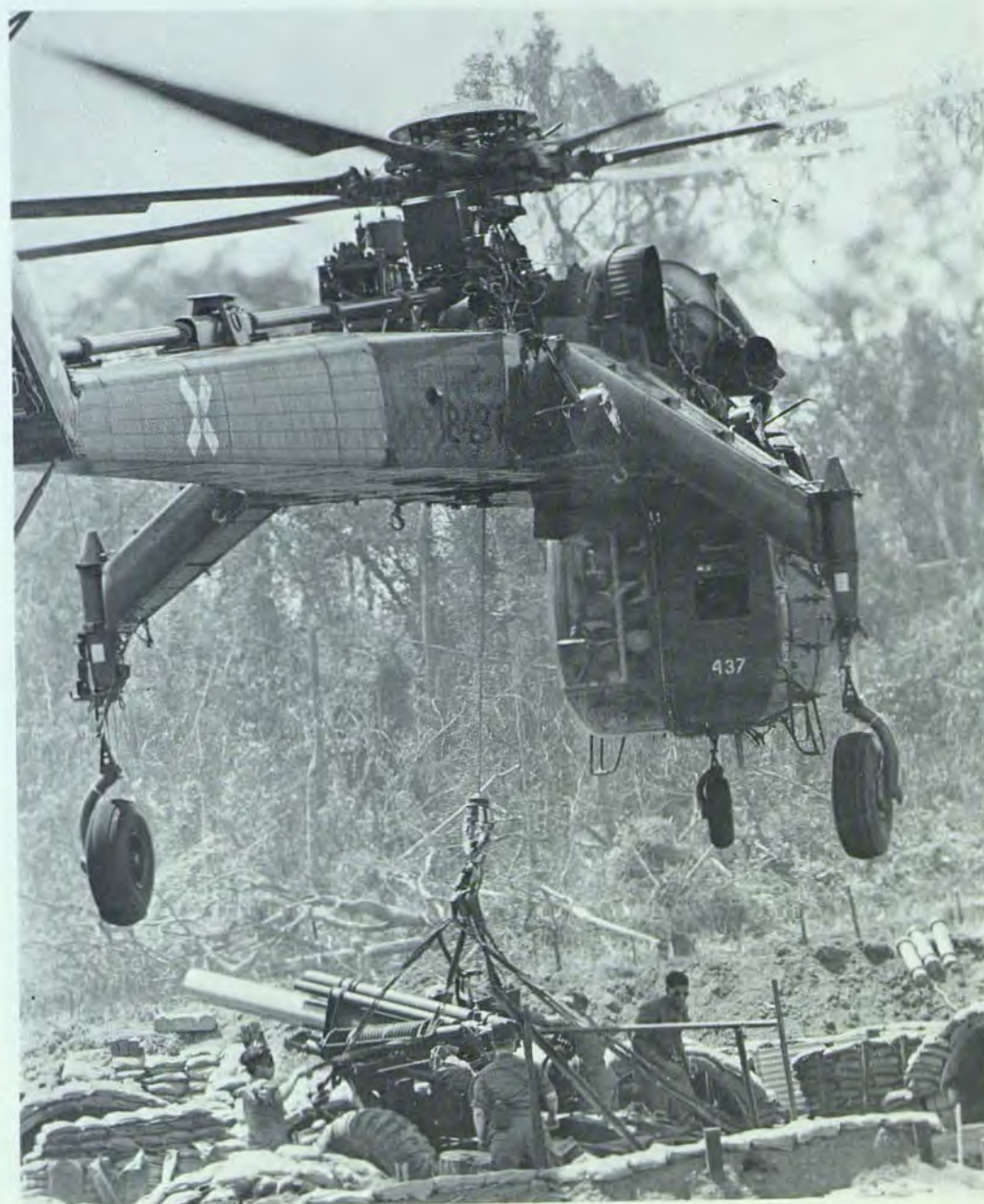
A newly emplaced 155 mm howitzer of the 1st of the 30th sits ready to lend high explosive support from a firebase north of Tay Ninh City in III Corps, while its crew works to improve the gunpit. Bulldozers of the 8th Engineer Battalion have pushed a protective mound of dirt up around the gunpit, a circle of earth that will serve both as protection against shrapnel from enemy rockets and mortars that strike close to the gun, and also as a fighting wall where the gun crew can defend its position and howitzer should the enemy penetrate the firebase.
