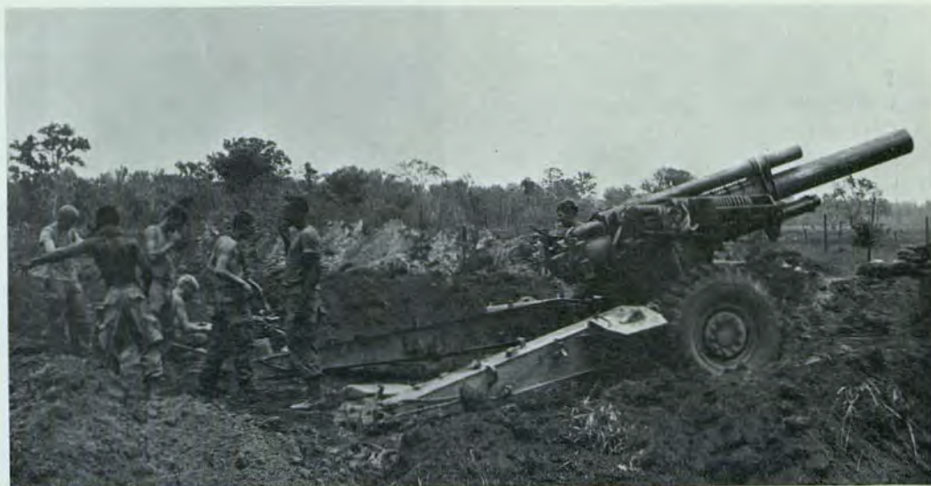
A newly emplaced 155 mm howitzer of the 1st of the 30th sits ready to lend high explosive support from a firebase north of Tay Ninh City in III Corps, while its crew works to improve the gunpit. Bulldozers of the 8th Engineer Battalion have pushed a protective mound of dirt up around the gunpit, a circle of earth that will serve both as protection against shrapnel from enemy rockets and mortars that strike close to the gun, and also as a fighting wall where the gun crew can defend its position and howitzer should the enemy penetrate the firebase.
