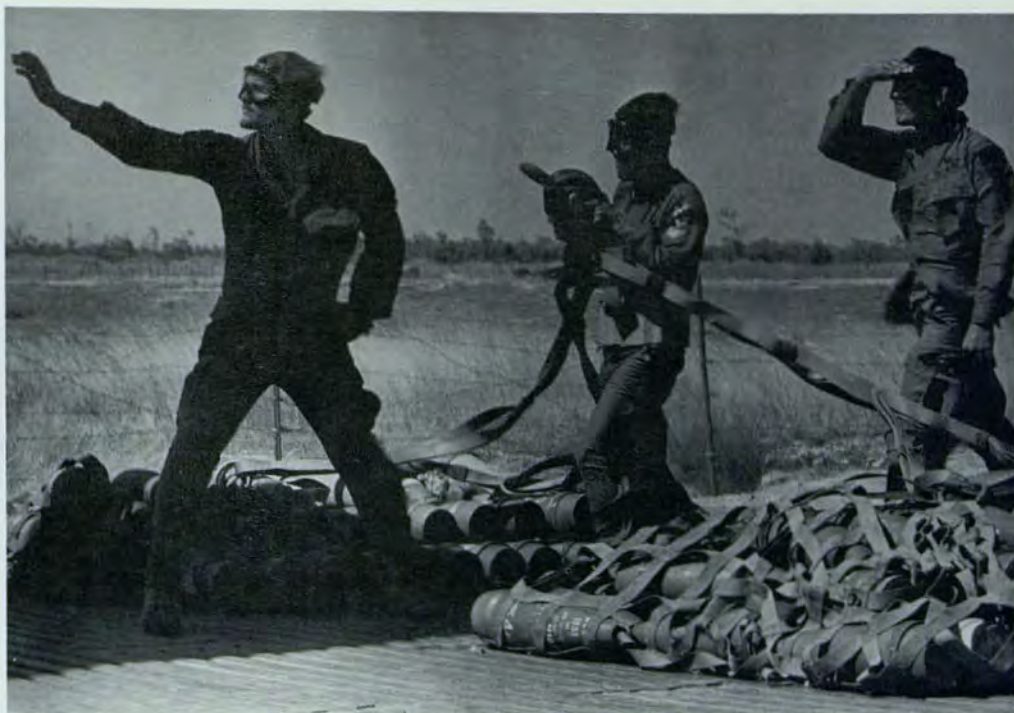
In late 1969 the 15th S&S riggers took part in a facet of Vietnamization, the Dong Tien or "Forward Together" program, when they taught ARVN troops, notably of the 1st ARVN Airborne Division, how to rig and sling out artillery pieces when using the CH-54 Flying Crane. While the ARVN student (top) holds the "doughnut," a 1st Cav Redhat at left keeps his hand forward to catch and ward off the approaching hook, a swinging hazard in the gale-force rotor wash of the giant helicopter.
