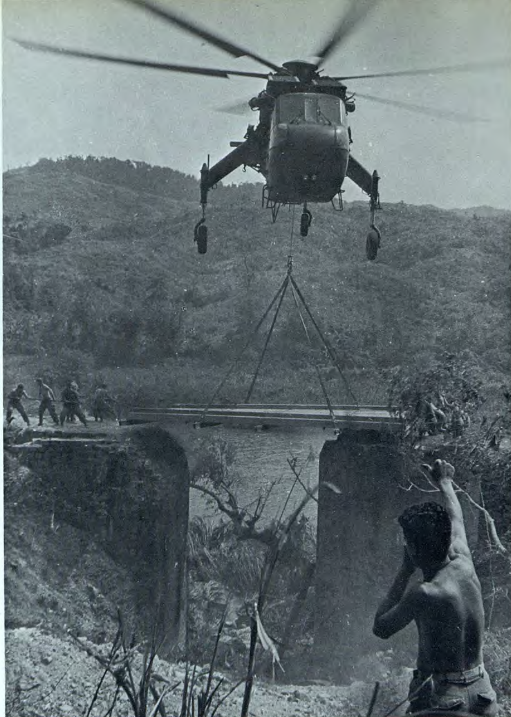
A huge CH-54 Flying Crane lowers a steel and plank bridge span into place as the 8th Engineers reopen another section of Highway 9—the only ground route into the besieged Marine base at Khe Sanh—during Operation PEGASUS, the relief of Khe Sanh.
