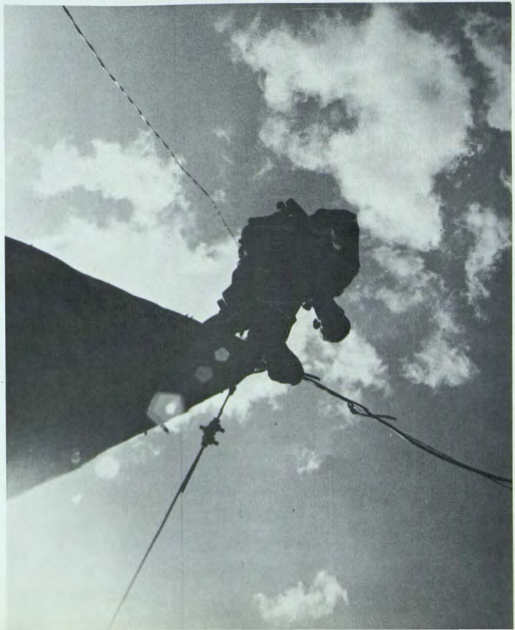
A cameraman with an artist's eye caught this signalman high on a commo pole, as he worked to string more telephone wire in an ever increasing communications network.
