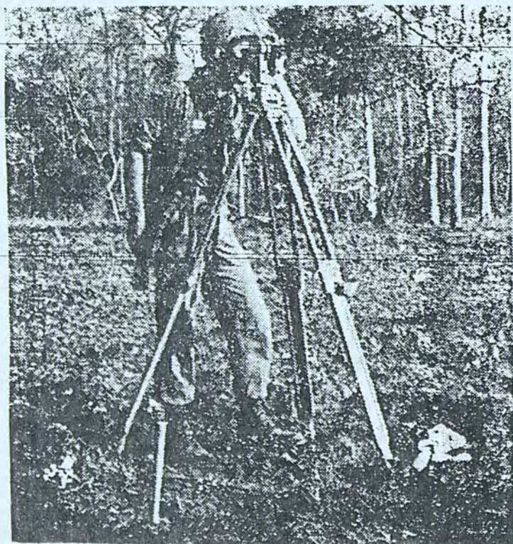
SIGHTING IN —Private First Class John H. Forsythe, of the 168th Engineer Battalion, surveys the area where his unit built an airstrip during Operation Junction City. (Photo by 168th ENGR-10)
