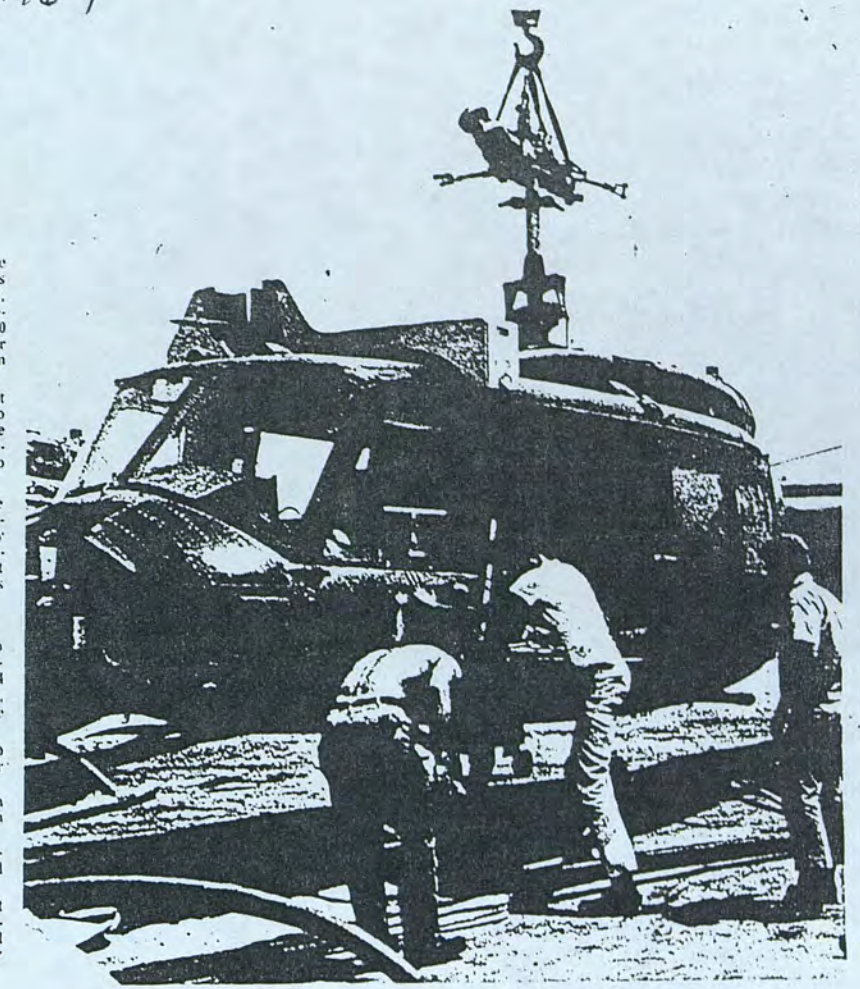
New landing skids are emplaced for easy shipment.
