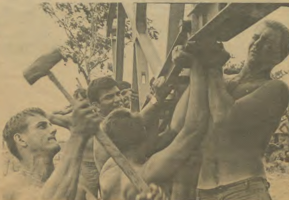
As a group of engineers holds the panel in position, SP5 Richerson drives the pin into place.
