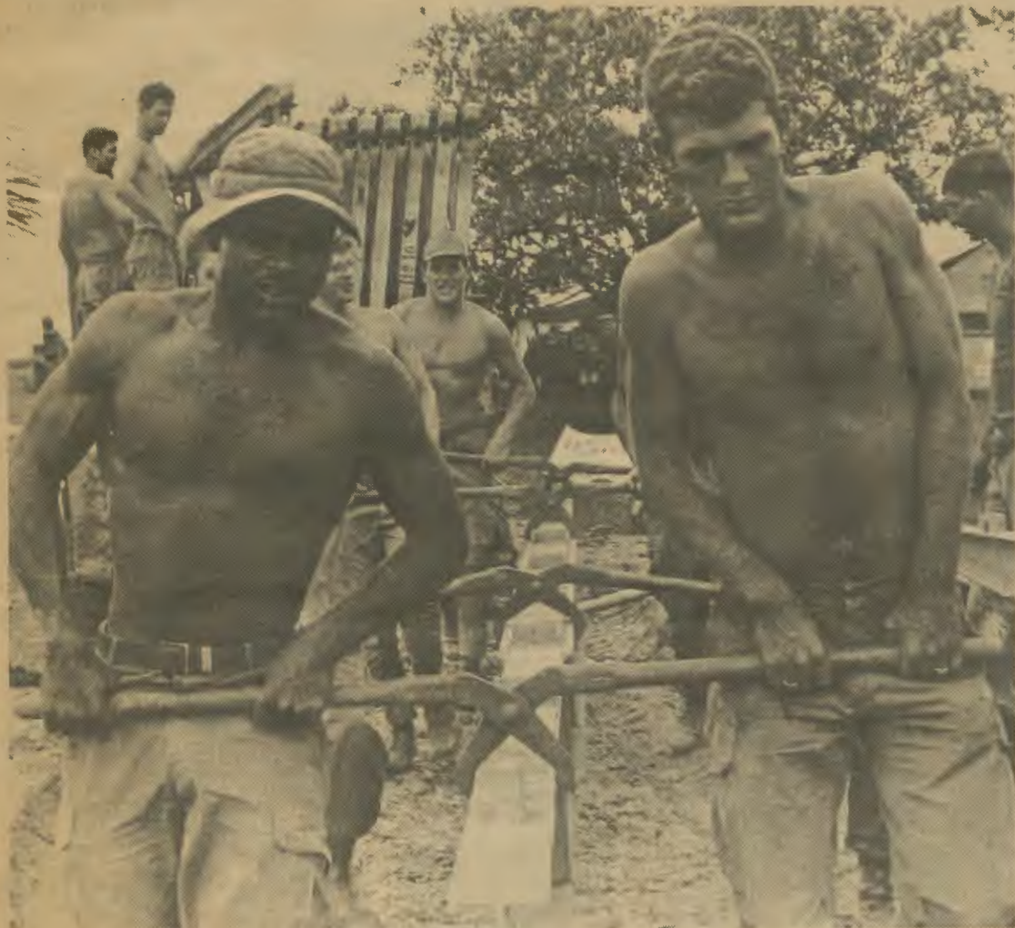
SP4 Melvin Wilkerson (left) and SGT John Bilton lead a transom out to the Bailey Bridge.
