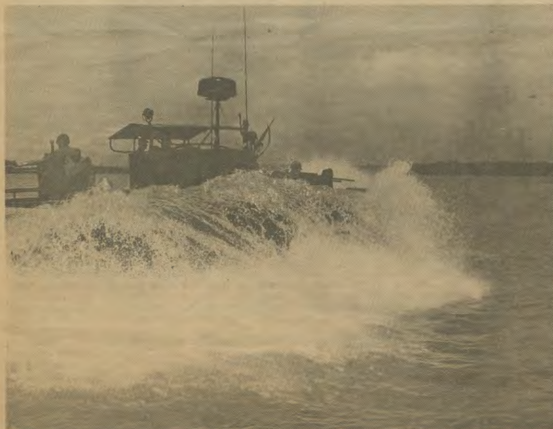
PBR executes a 180 degree turn in one boat-length while traveling at top speed: 32 knots.
