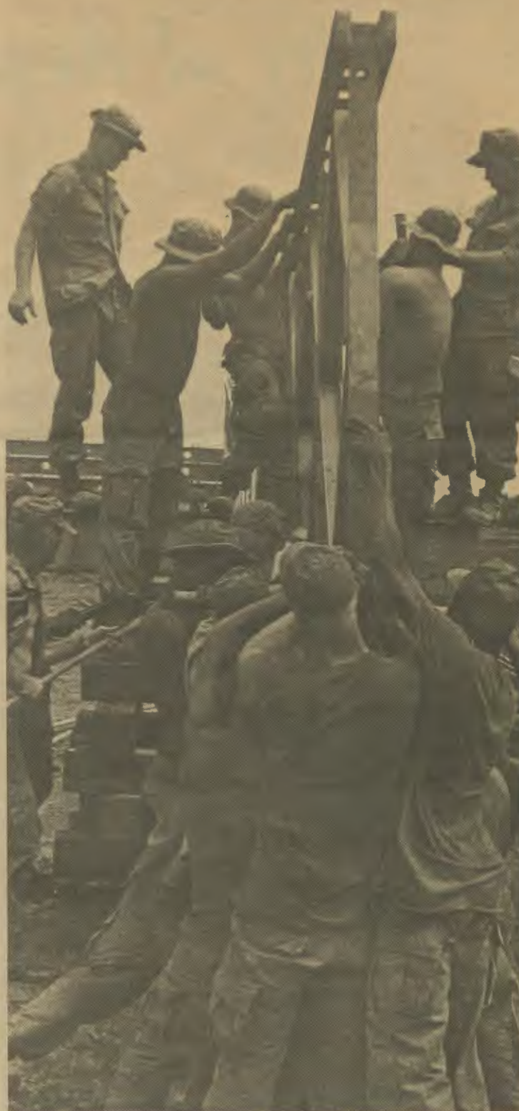
Engineers from the 15th Engineer Company (Provisional) work as a precision team to position a panel for the Bailey Bridge.
