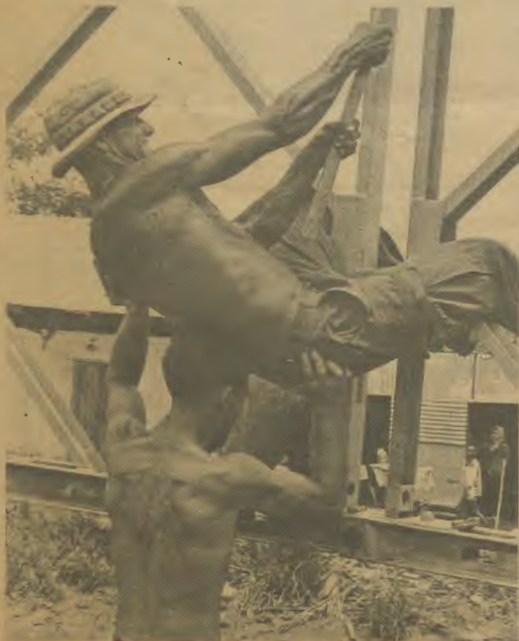
SP5 David Richerson gets a boost as he drives a pin into a bridge panel.
