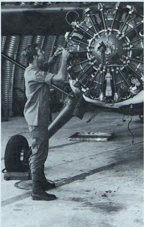
*A check is made of the engine safety wiring prior to the placement of the propeller.*
