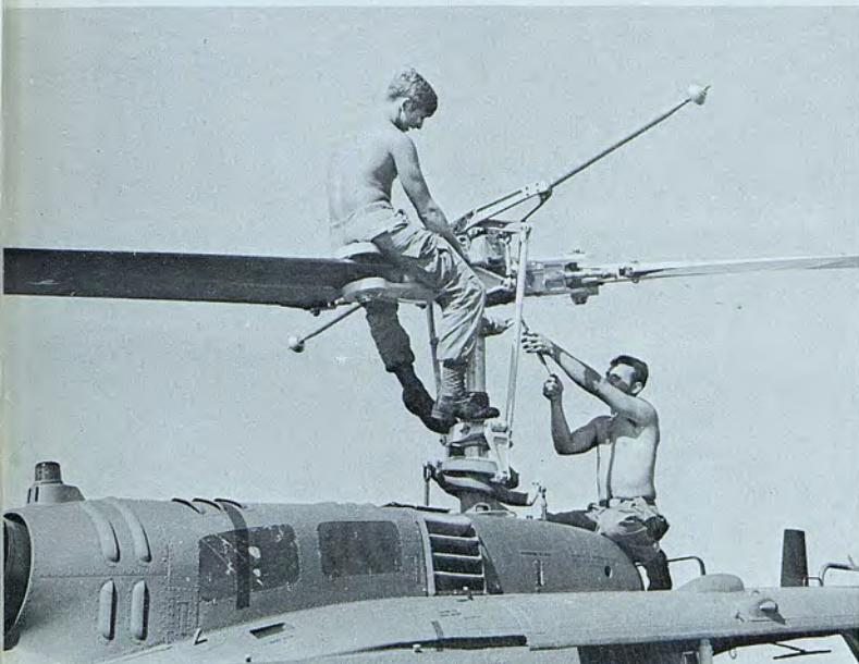
*Mechanics from the 610th Transportation Company safety wire a Huey rotor head.*
