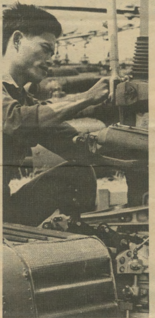
VNAF mechanics continually check their aircraft's rotor-drive assemblies. Both the 211th and the 217th squadrons recently switched over to new turbine-powered rotor craft from their older piston-engined types.
