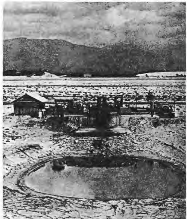
Called Phantom Lake by base personnel, rain-filled hole is caused by jet engine blasts at Cam Ranh Bay jet engine test cell operation site.
