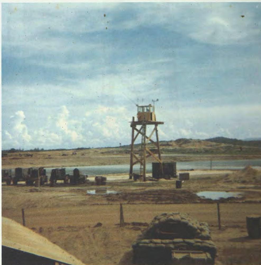
Control Tower at LZ Baldy late 1969. (Chet Newcomb photo.)
