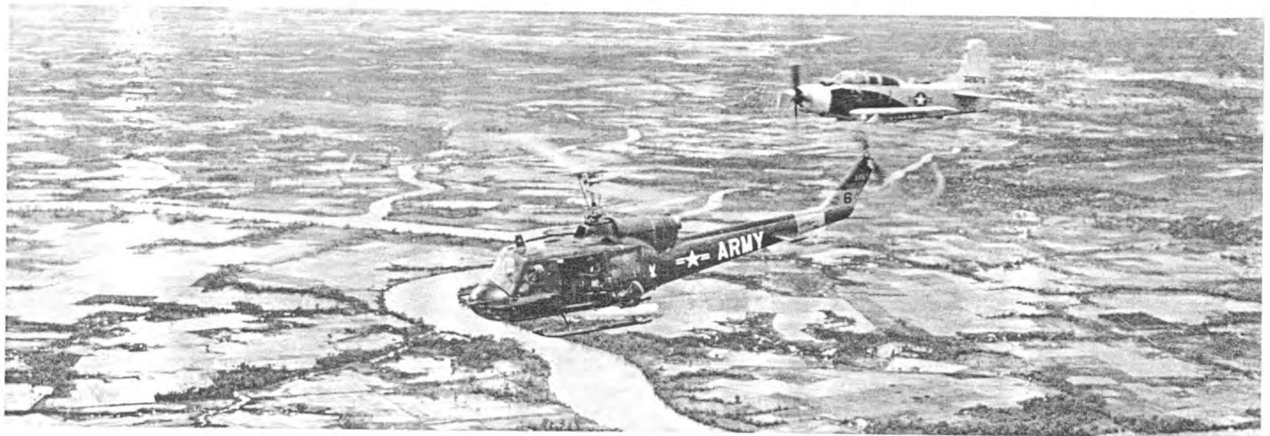
Army UH-1B and Air Force A-1E Skyraider worked as "Hunter-Killer" Team in South Vietnam, 1964. Huey is armed with quad .30 cal MG and M157 rocket pods, and carries old gloss OD finish. "ARMY" on fuselage in white, yellow tail markings, white eagle on nose and fuselage.
