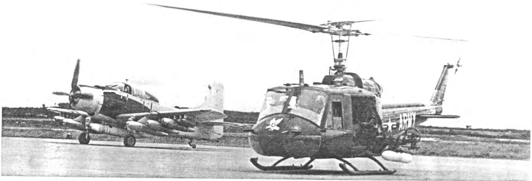
Army UH-1B and Air Force A-1E Skyraider worked as "Hunter-Killer" Team in South Vietnam, 1964. Huey is armed with quad .30 cal MG and M157 rocket pods, and carries old gloss OD finish. "ARMY" on fuselage in white, yellow tail markings, white eagle on nose and fuselage.
