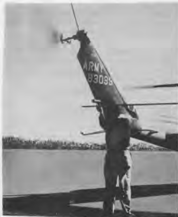
Figure 8-35. Tracking tail rotor blades (UH-1B Serial No. 60-3546 thru 64-14100)
