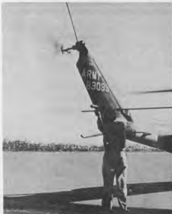
Figure 8-30. Tracking — tail rotor blades (UH-1A)
