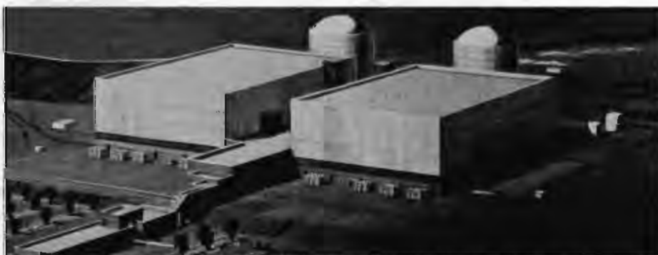
McGUIRE NUCLEAR STATION COWANS FORD, NORTH CAROLINA Duke Power Company Charlotte, North Carolina SUPREME and GILCO GROUTS USED THROUGHOUT
