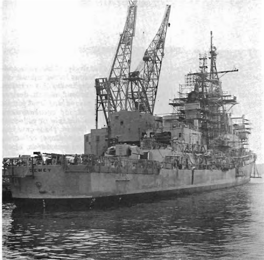
The DEWEY during modernization
