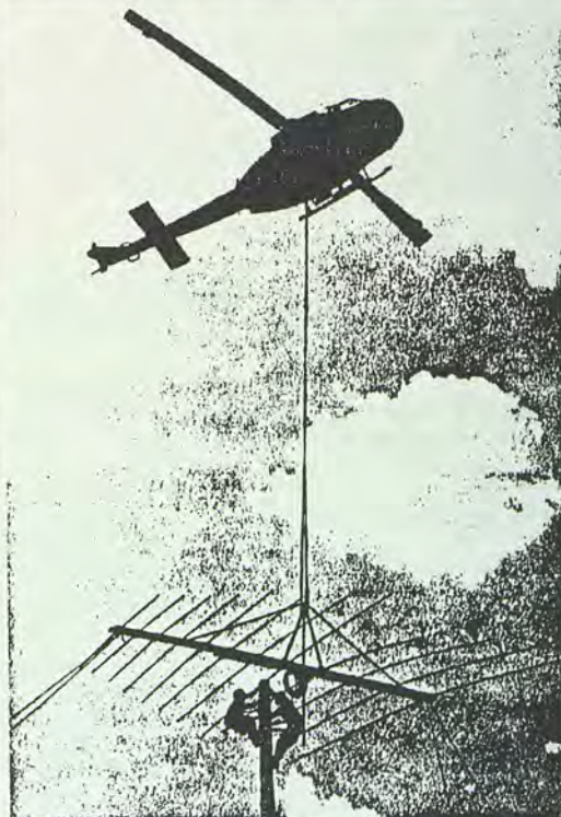
"A LITTLE HIGHER and to the left, please. That's it—easy does it." And that's how the Brigade's new "MARS" station got its 300-pound antenna on the 60-foot pole. (Photo by Fuller)
