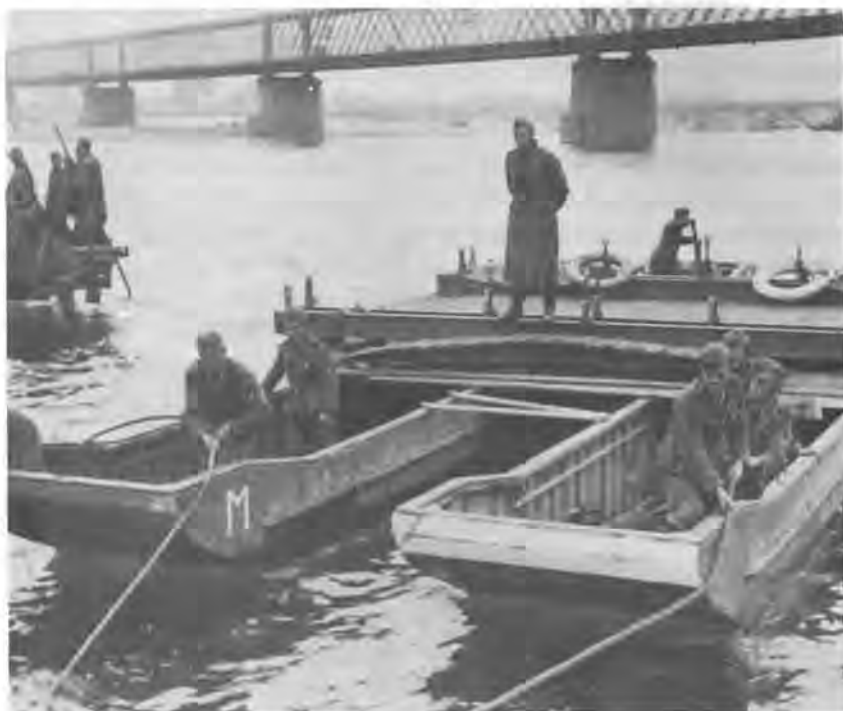
CONSTRUCTION of a German ponton bridge, 1941.
