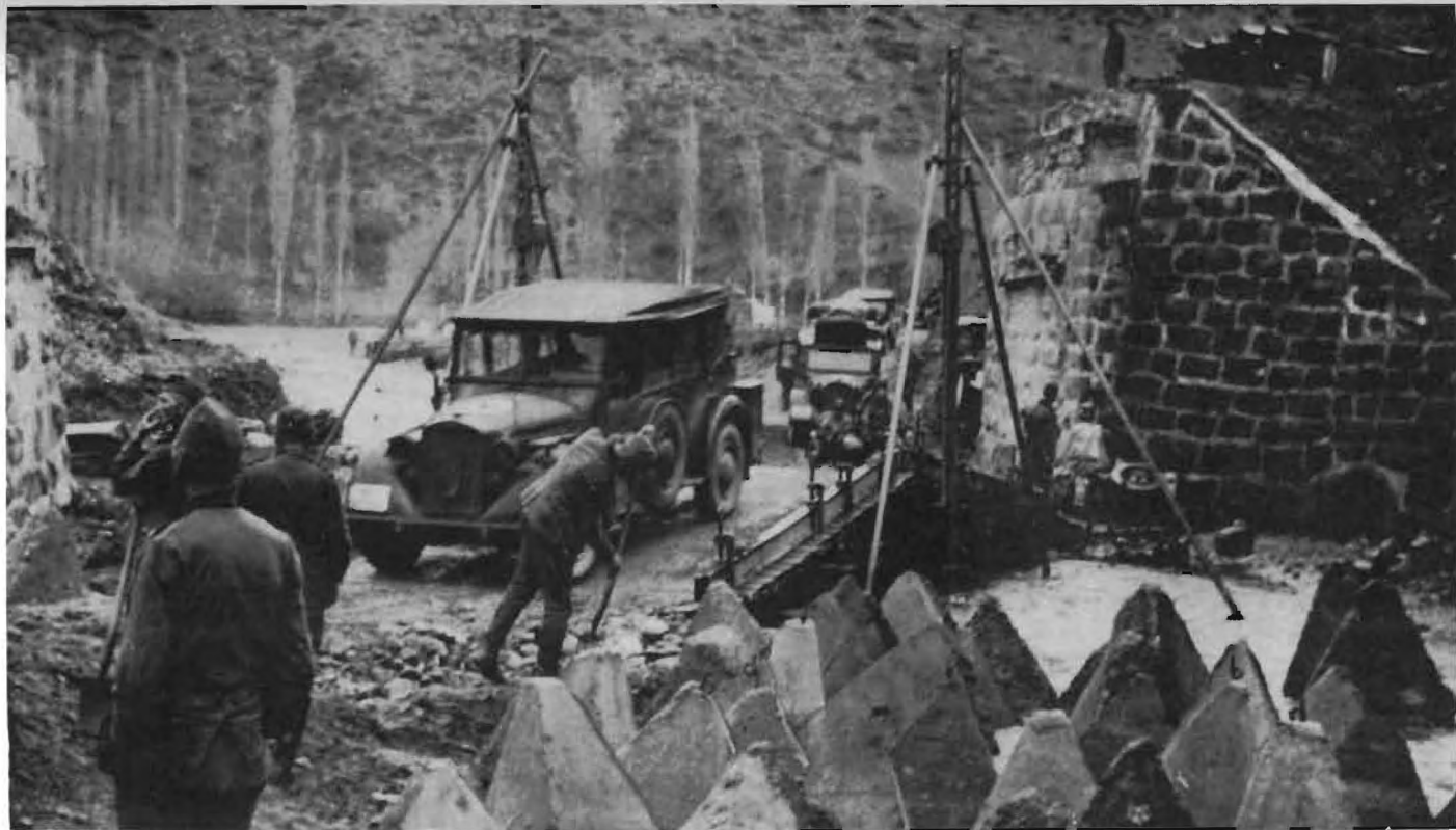
Figure 5. German emergency bridge replaces demolished structure.
