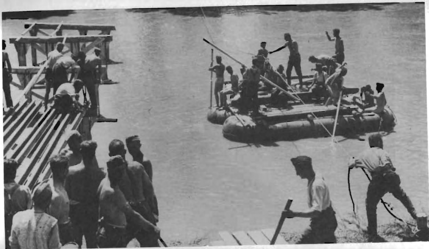
Figure 26. Construction of an emergency bridge near Thermopylae Pass.
