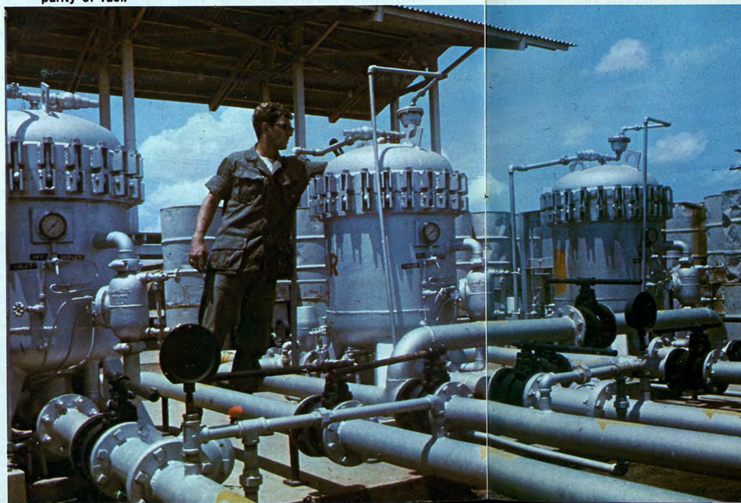
Separators filter out sediment, solids, and water to insure purity of fuel.
