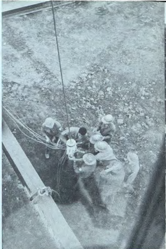
ARVN engineers attach the big hook to a 9,000 pound beam.
