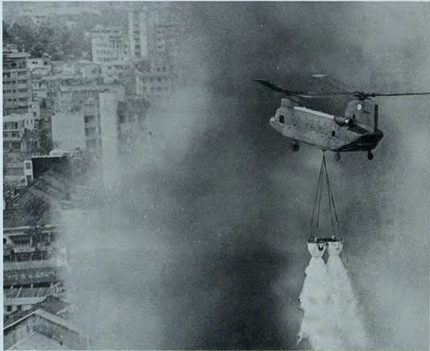
Chinook opens bucket doors and drops water onto fire as it flies through dense smoke from fire below.
