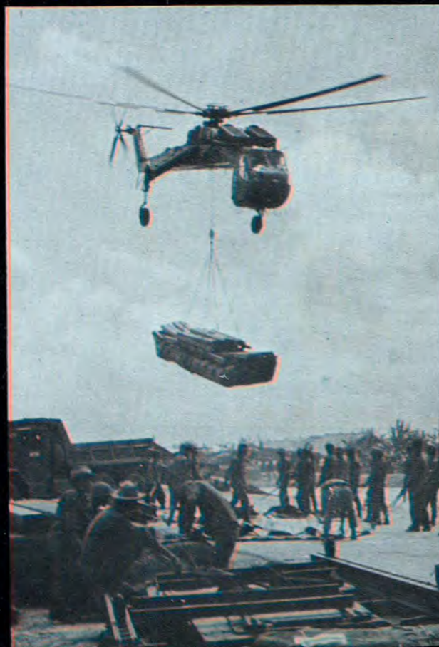
The pontoon bridge is to replace the old Rt. 4 bridge across the Van Co Dong River knocked out by V.C.
