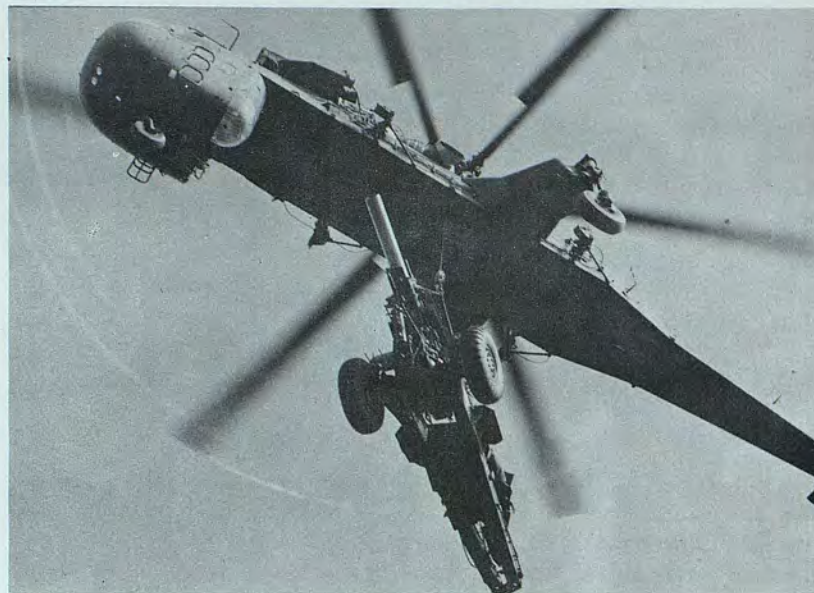
The large 155 mm howitzer—a typical load for a crane.
