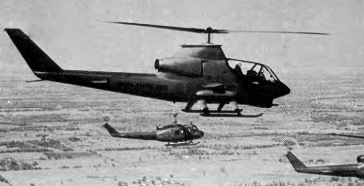
A HueyCobra gunship introduced in October 1967 flies alongside an older UH-1D. The chin turret is directed toward its target by the pilot turning his head. Photo by 1st Aviation Brigade—IO.
