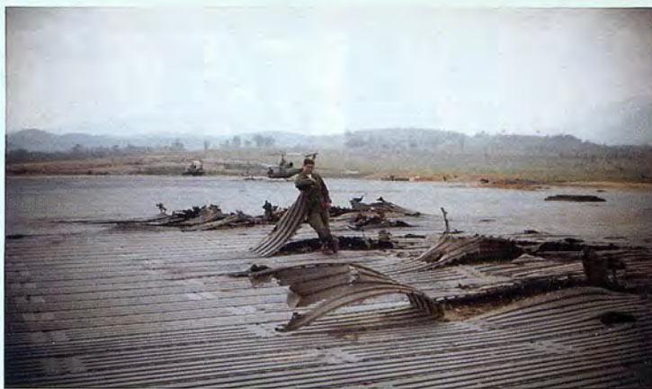
Mel poses with pieces of a PSP runway just west of Kontum damaged by direct mortar hits.
