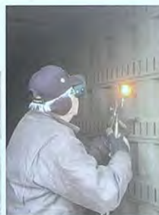
Gil Fluhr burning out holes for vents
