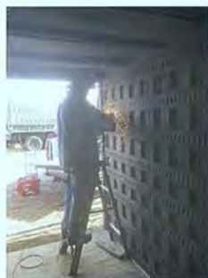
Marshall Eubanks making cuts for vents
