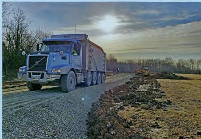
Two hundred foot gravel drive under construction.
