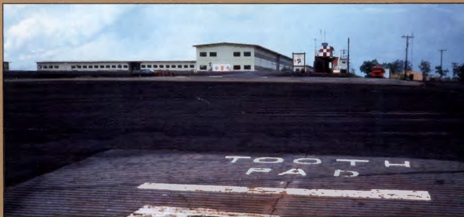
Pad 14 at Headshed Helipad, Long Binh, USARV Headquarters, April 1971.
