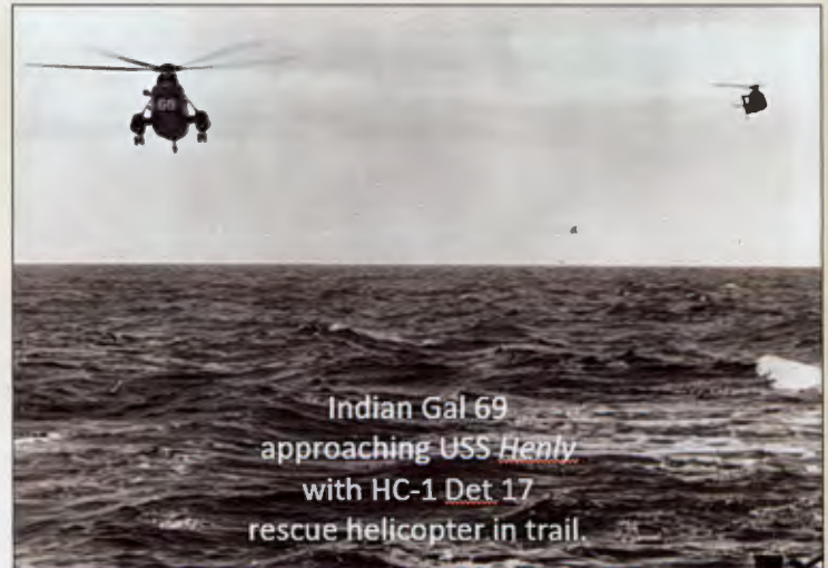
Ditching following tail rotor control cable loss due to battle damage
