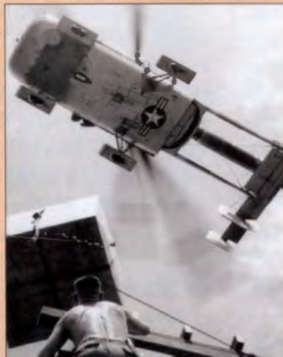
HH-43B 62-4565 helping build a shower at NKP 1064.
