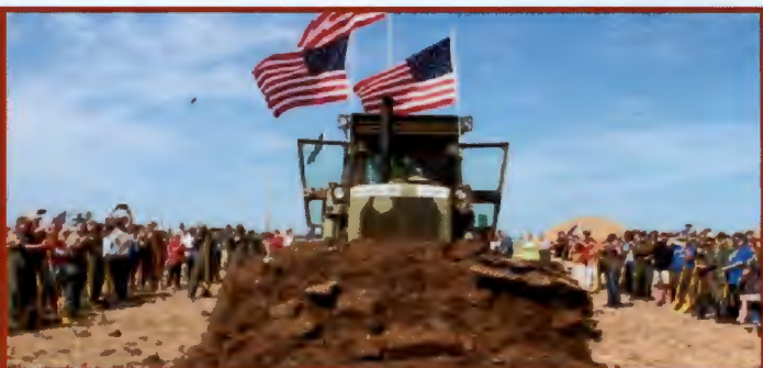
Grading for the brick sidewalk
