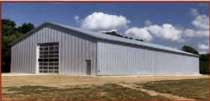
60' x 140' storage building @ NW corner
